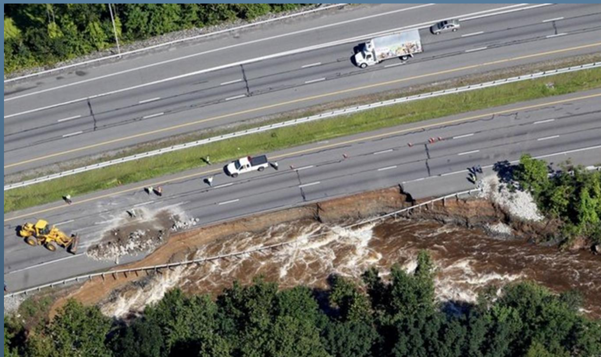
Route 287 in Morris County – Northbound shoulder washed away by floodwaters from Hurricane Irene
